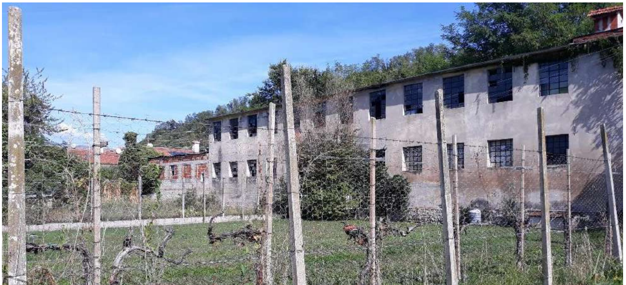
Figure 5. Former Gioppo Textile Factories at Montebelluna, view of the façade of the first building to the west, current condition
