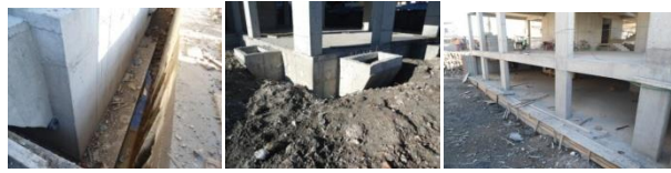
Figure. 3.2.1: The foundation of the project
