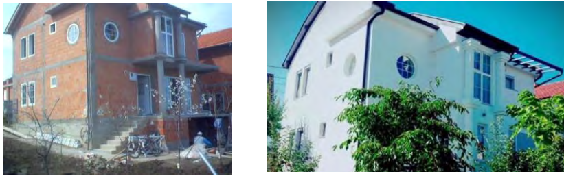
Figure 1. Home of the Qerimi family before and after the intervention (Qerimi, 2019)
