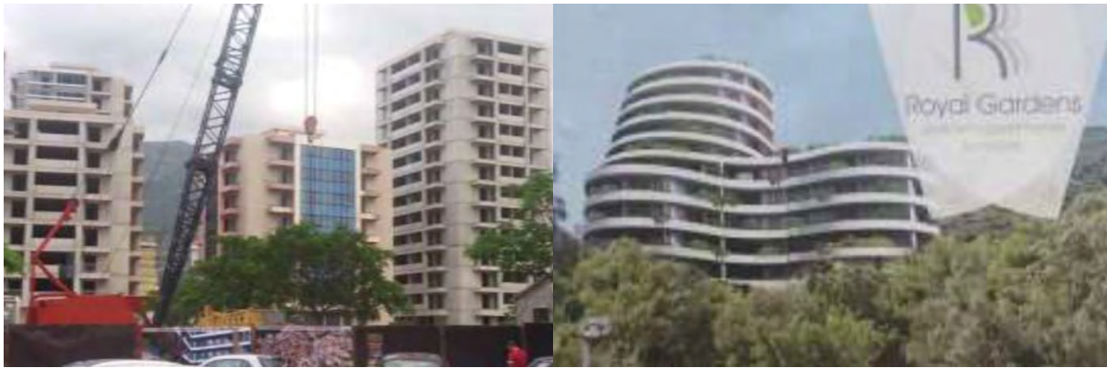
Figure 3. Budva, buildings under construction, 2017.
