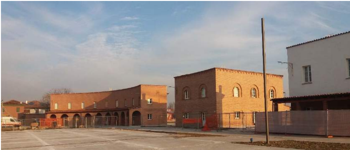
Figure 14. The rural houses in Vigonza at the end of the restoration transformation, view of the first buildings from the east (November 2015). The façades on the piazza are made of exposed brick with the exclusion of the corresponding portion on the upper floor of the building with convex trend (on the right, partially off).
