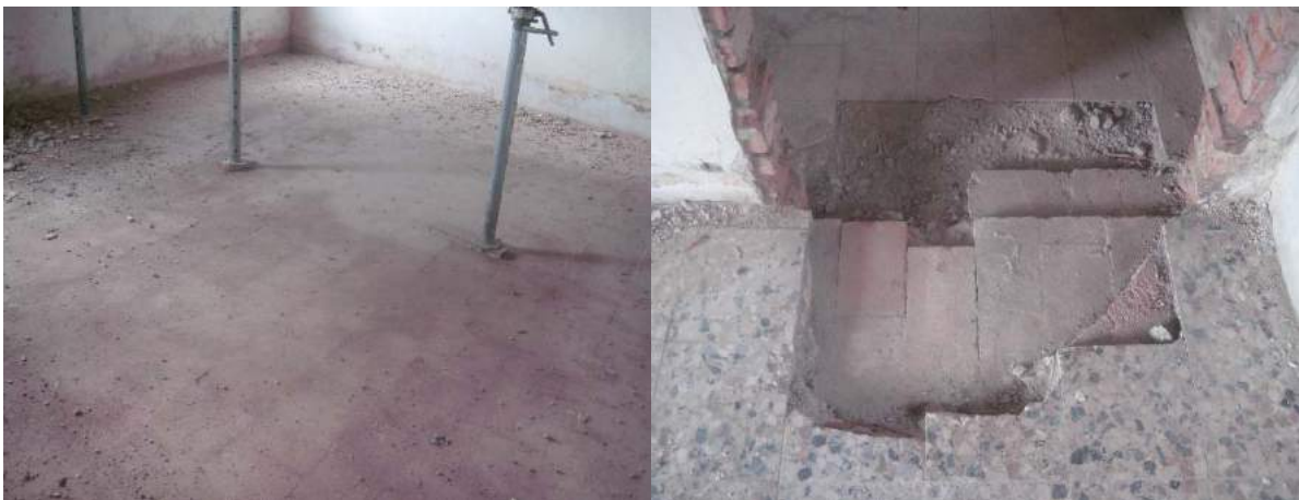
Figures 9, 10. The rural houses that close off the southern side of the new piazza in Vigonza (1937-1938). Ground floor, the original floor of terracotta square tiles, laid without joints simulating continuous flooring (preliminary phase of the restoration, 2012-2013).
