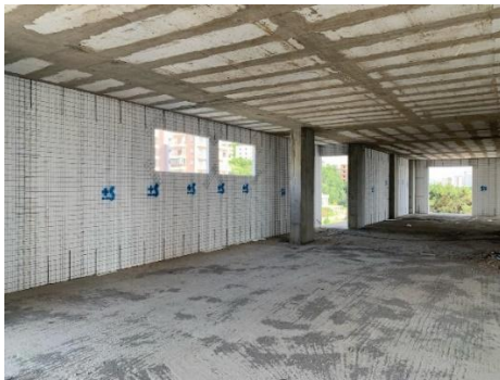
Fig. 2+3. Internal and external walls with polystyrene panels reinforced with iron brackets (Photo by the authors)
