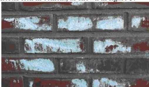
Fig. 5. The phenomenon of the creation of mold and the accumulation of salts in the brick wall (from "Building materials" book, F. Kadiu)
