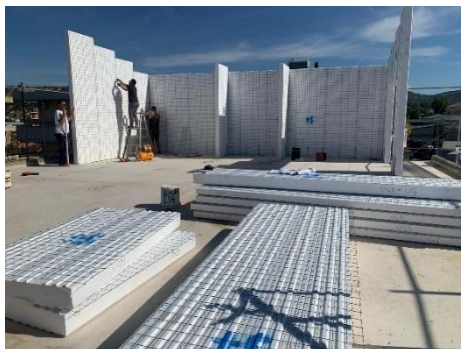
Fig. 6. Polystyrene panels reinforced with galvanized iron bars (Photo on site by the authors)
