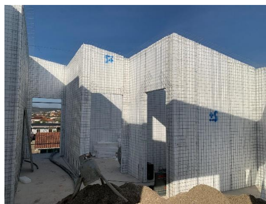
b. Realization of internal walls
