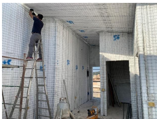
a. Realization of internal walls and soles
