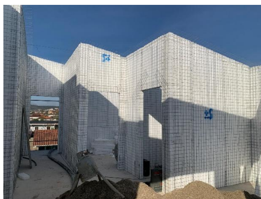
b. Realization of internal walls
