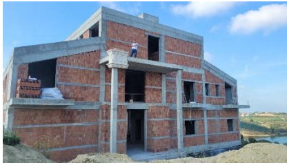
Fig 1. B/A frame building with infill masonry with lightweight bricks
