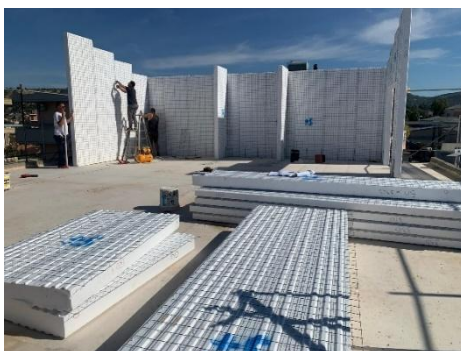
Fig. 6. Polystyrene panels reinforced with galvanized iron bars (Photo on site by the authors)
